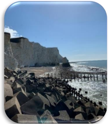
Tetra pod sea defences on the south coast
